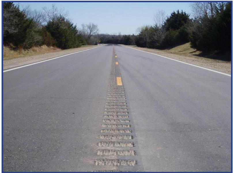
**Figure 1. Centerline Rumble Strips in Kansas**
